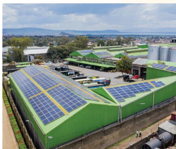
Aerial view of the 850 kW rooftop system.
