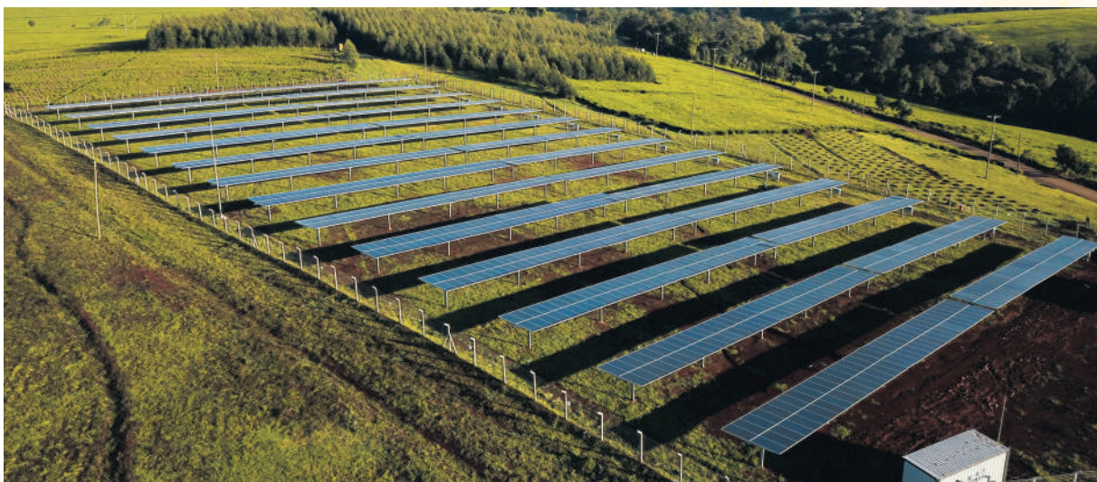
JAMJI solar power plant, Kericho, Kenya, with trackers in stow position.
